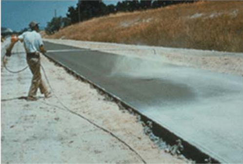
Liquid membrane-forming compounds sprayed onto the surface are effective, economical moisture barriers for moist-curing concrete.
