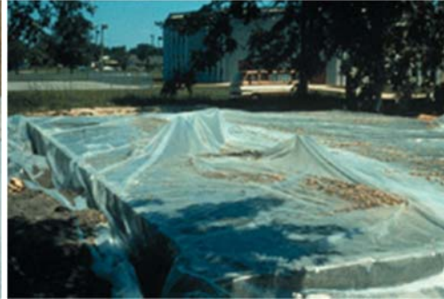
Polyethylene sheets are effective, economical moisture barriers for moist-curing concrete.
