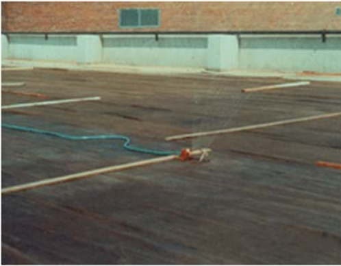
Burlap kept saturated with water is an effective medium for moist-curing concrete.
