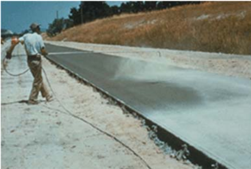
Liquid membrane-forming compounds sprayed onto the surface are effective, economical moisture barriers for moist-curing concrete.
