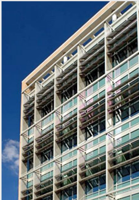
The stepped design at CDC Building 110 Facility provides overhangs and light shelves to shade and direct natural light into the office spaces inside.
