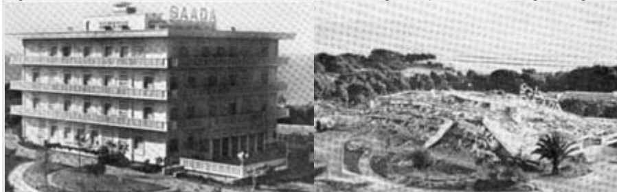
Fig. 3. Left : Saada Hotel (before)—Agadir, Morocco, 1960 and Right : Saada Hotel (after) ground shaking damage—Agadir, Morocco, 1960
