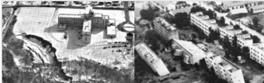
Fig. 2. Left : Ground failure-landslide—Alaska, 1964 and Right : Liquefaction damage—Niigata, Japan 1964
