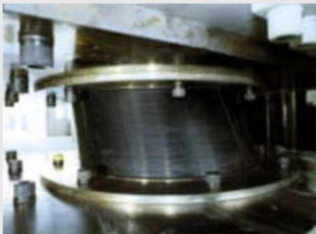
Fig. 9. Base Isolation Bearings are used to modify the transmission of the forces from the ground to the building
