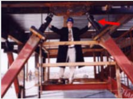
Fig. 10. Passive Energy Dissipation includes the introduction of devices such as dampers to dissipate earthquake energy producing friction or deformation.
