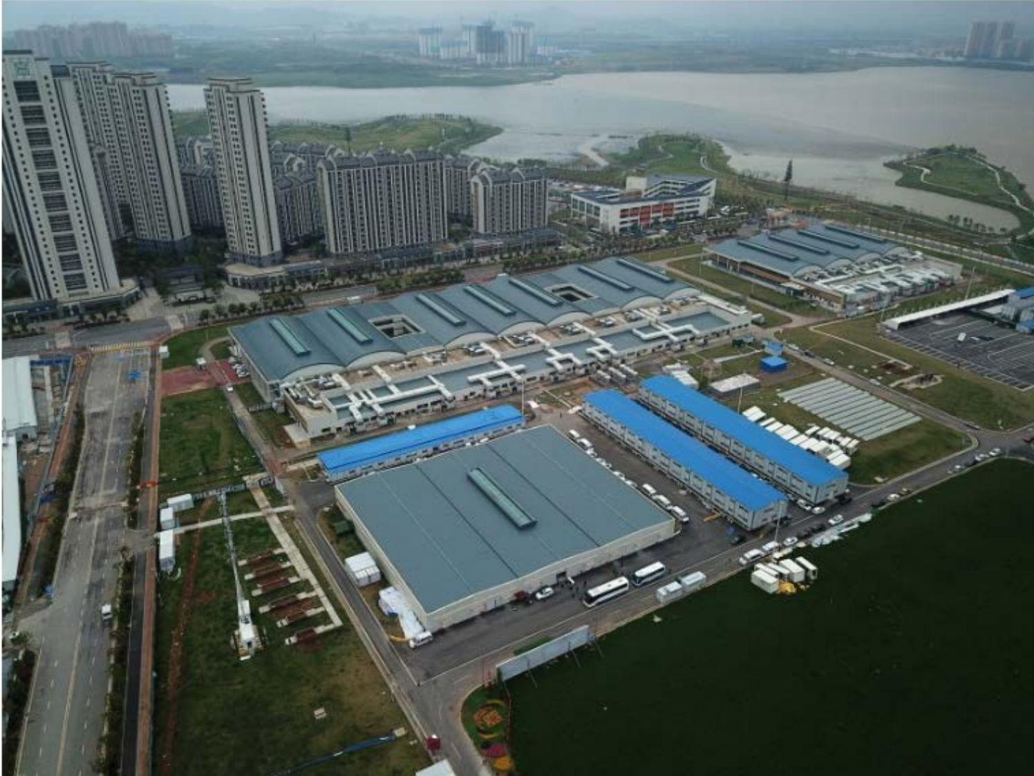
Leishenshan Hospital was constructed on a parking lot from prefabricated modules in two weeks in Wuhan, China. (Sam McNeil / Associated Press)
